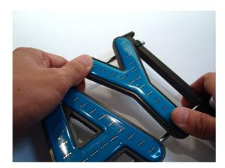
E3. Then align and fasten the top clips onto the top Stainless Steel Rod. Make adjustments in spacing as you see fit.
